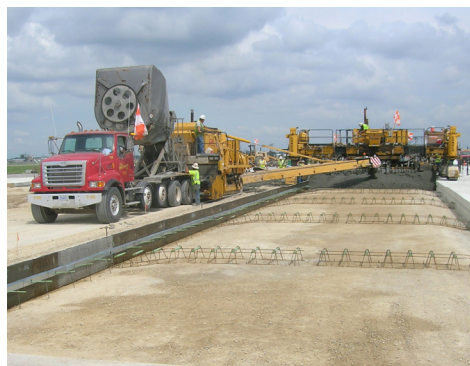
Crews constructing the Taxiway C extension
