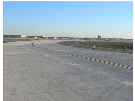
The finished Taxiway C extension
